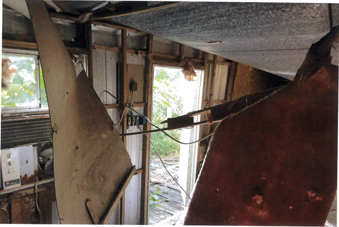
LIVING ROOM LOOKING AT FRONT DOOR
