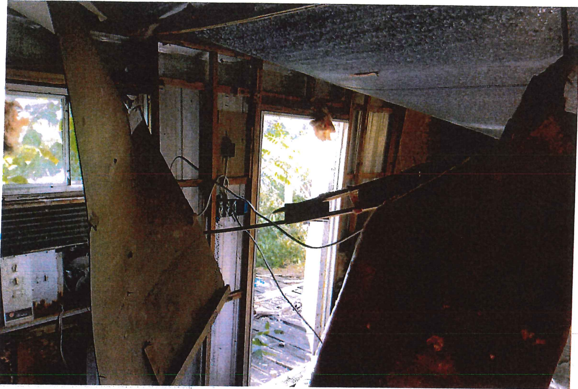
LIVING ROOM LOOKING AT FRONT DOOR
